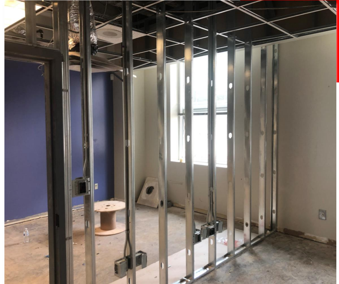
Metal Stud Framing in New Admin Suite in C. Allen Building
