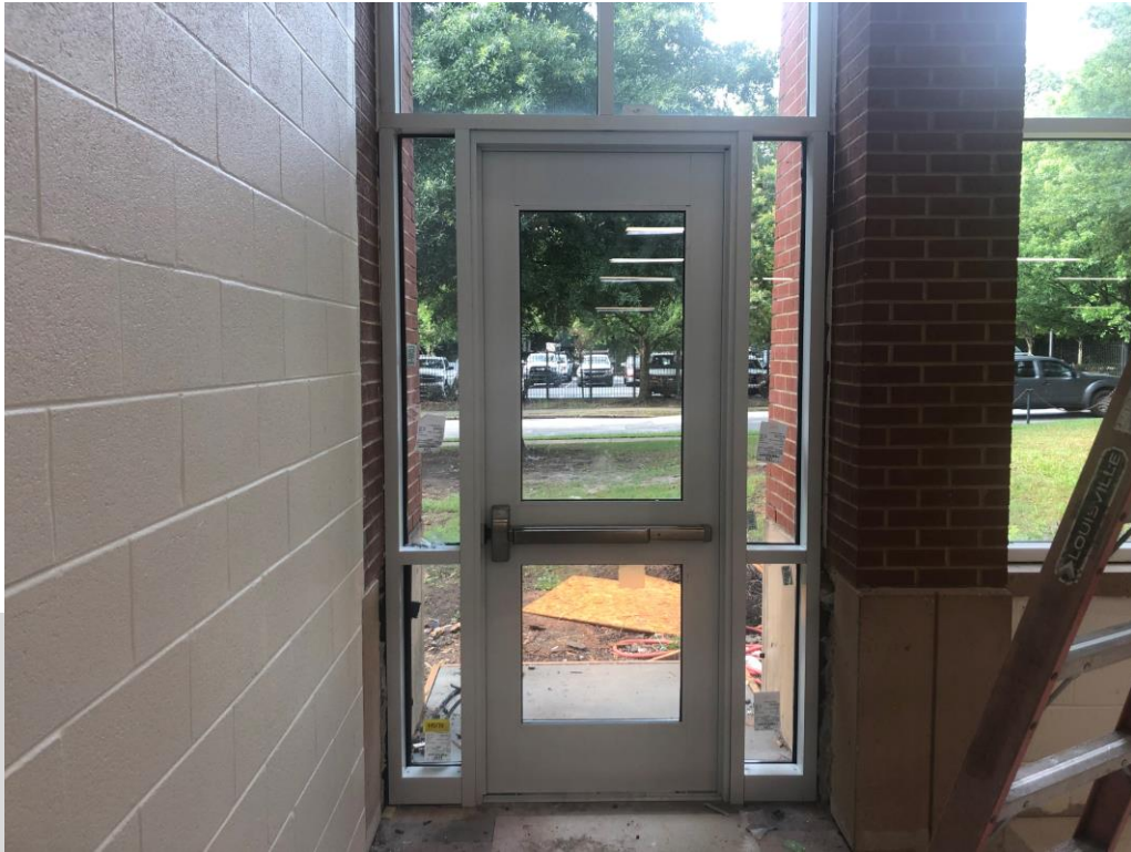
Storefront Door Installed in 8 th Street Multipurpose Room
